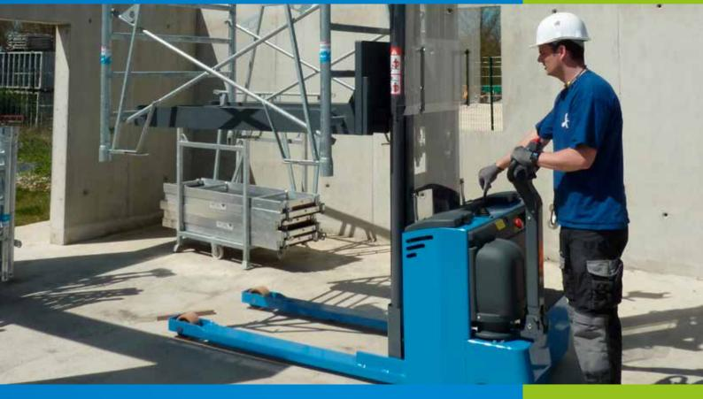
The Monte-Tour system offers a revolutionary tower assembly method, in the opposite direction from traditional assembly. This removes the risks of falls from height and falling objects.
