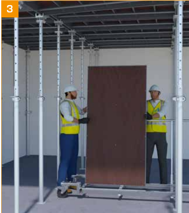
3 - Store the panels on the wheeled base so they can be moved easily to the next cell.
