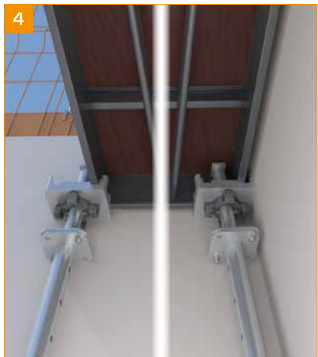
- The prop in the corner of the cell must be pressed perfectly flat against the skin.
