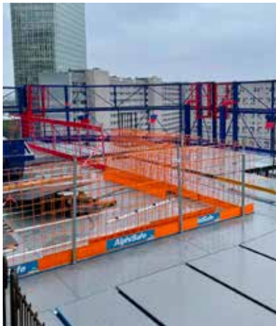
Intermediate safety allowing formwork installation to continue
