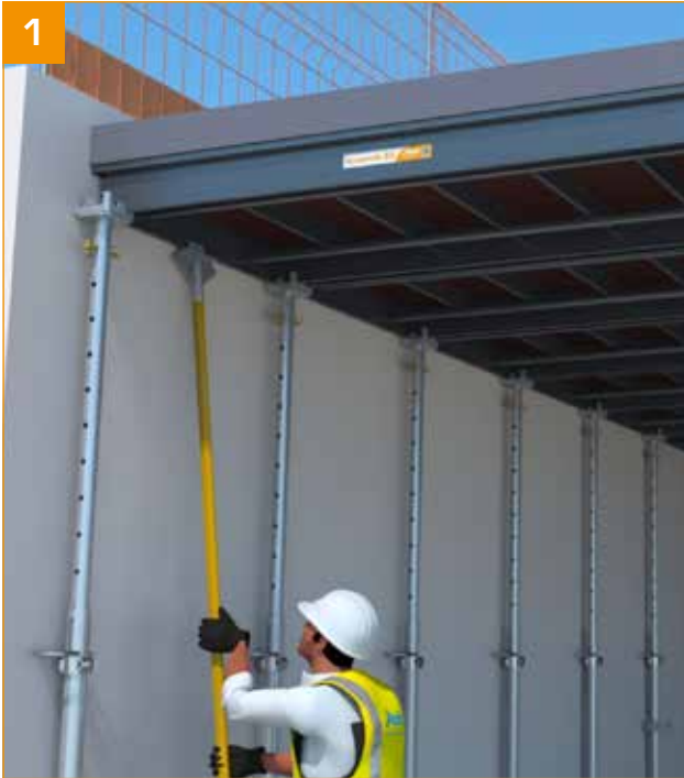
1 - At the start of a frame, position the HorizontalAL pole at the centre of the first panel.
