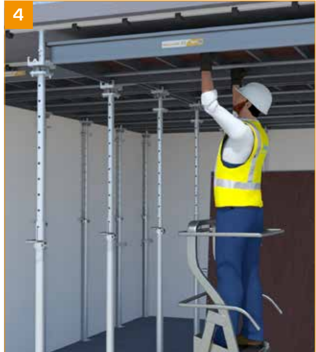
4 - For the rest of the cell, strike down the quick-removal heads. - Shift the panel horizontally so you can tilt it.
