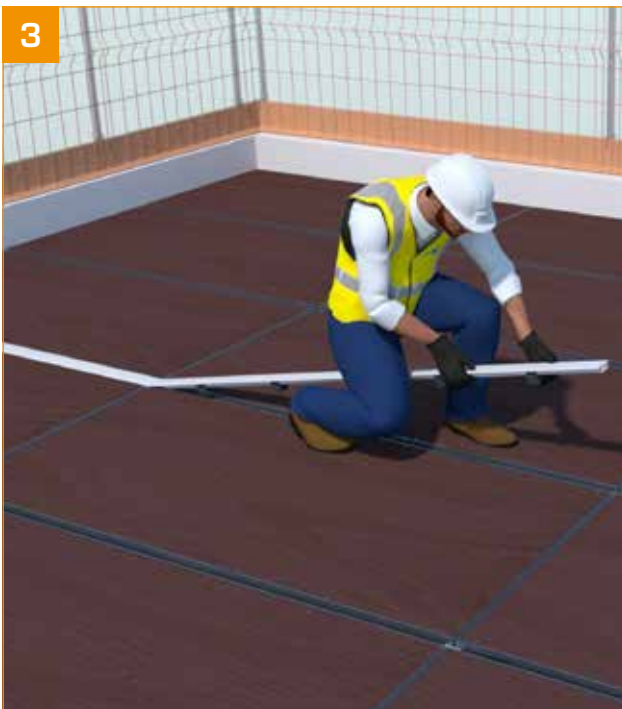
3 - Install the seal by clicking it in place between two panels.
