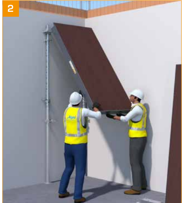
- Attach the first panel.
