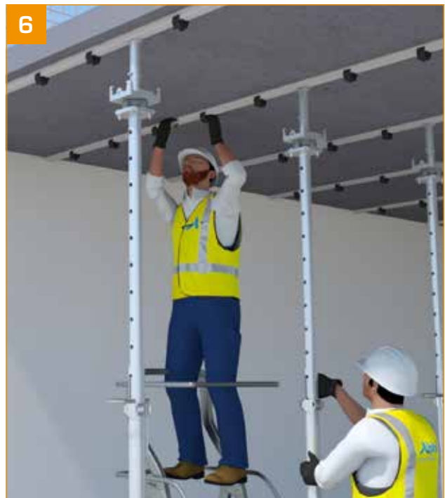
6 - After drying, remove the seals and props.
