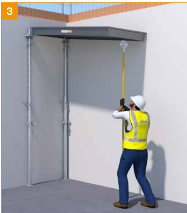
- Raise the panel using the HorizontalAL pole.
